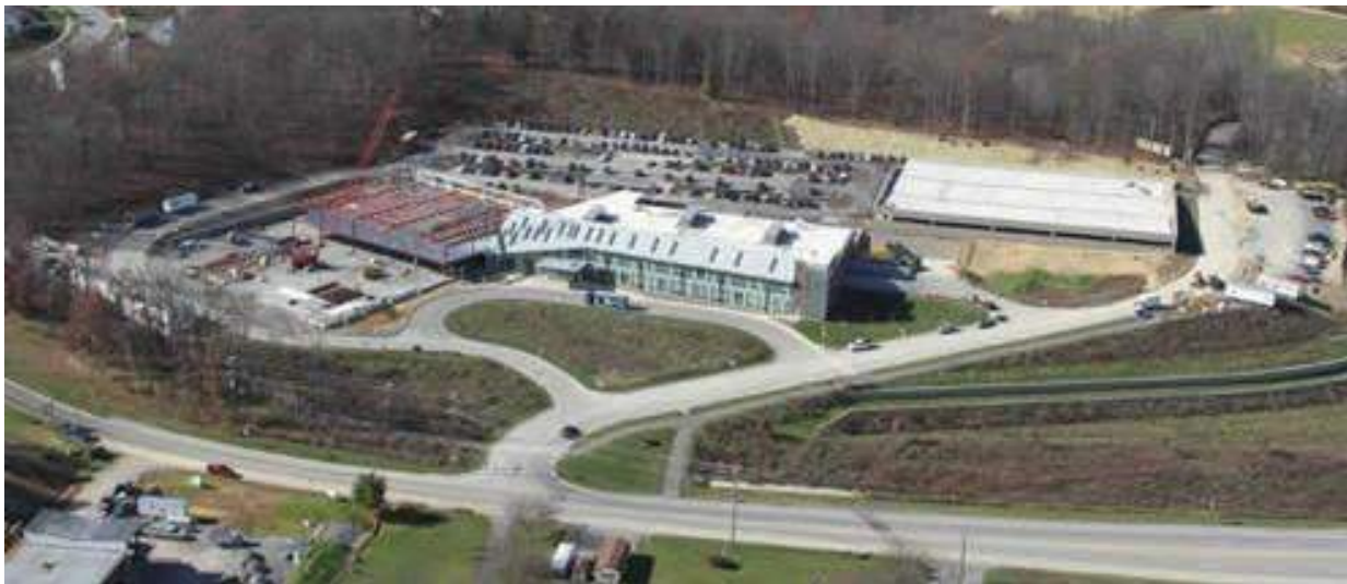
Figure 1.3: Aerial View of the Geisinger Grays Woods Ambulatory Care Campus. Image courtesy of www.pahomepage.com
